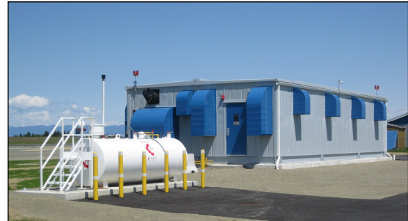
Fig. 1 24' x 46' Building divided into Regulator Room, Generator Room and Workshop, c/w 350 KW Prime Power Rated Diesel Generator, 14 Switchgear Regulators, 10 Non-Regulated Cells and Novec-1230 Fire Suppression System.
