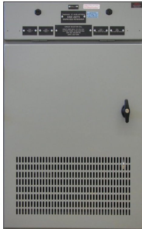
Fig. 1 L-847-4 Circuit Selector in 24" wide cell.
